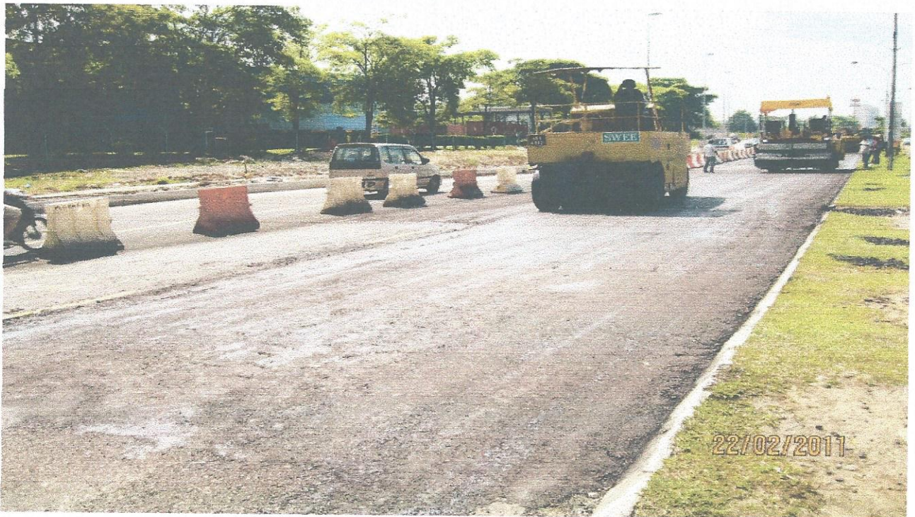
Photo 8 : Compacting Surface
