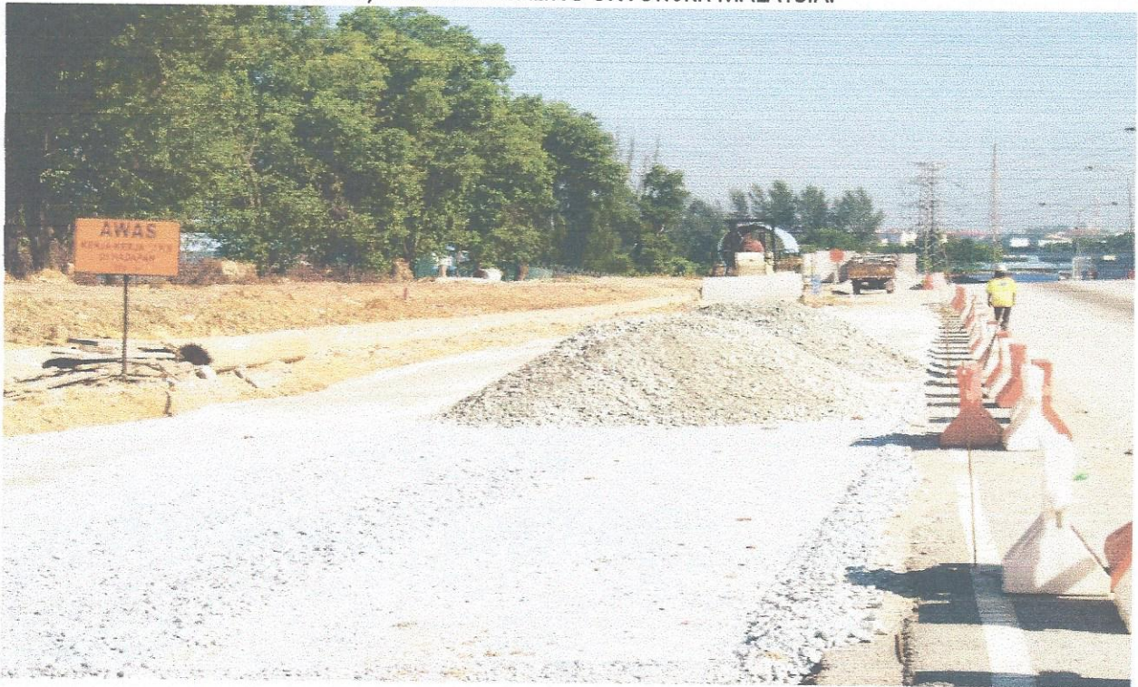
Photo 1 : Laying Crusher Run
